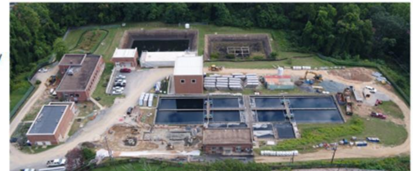
Raw Water Heat Recovery
