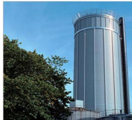
Thermal Energy Storage
