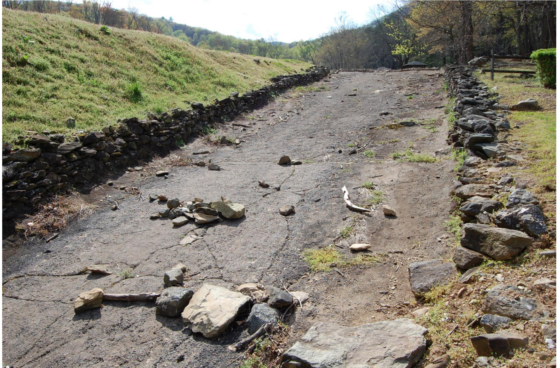
(Proposed) Mint Springs Valley Park Dam Improvements – 2023-2024
