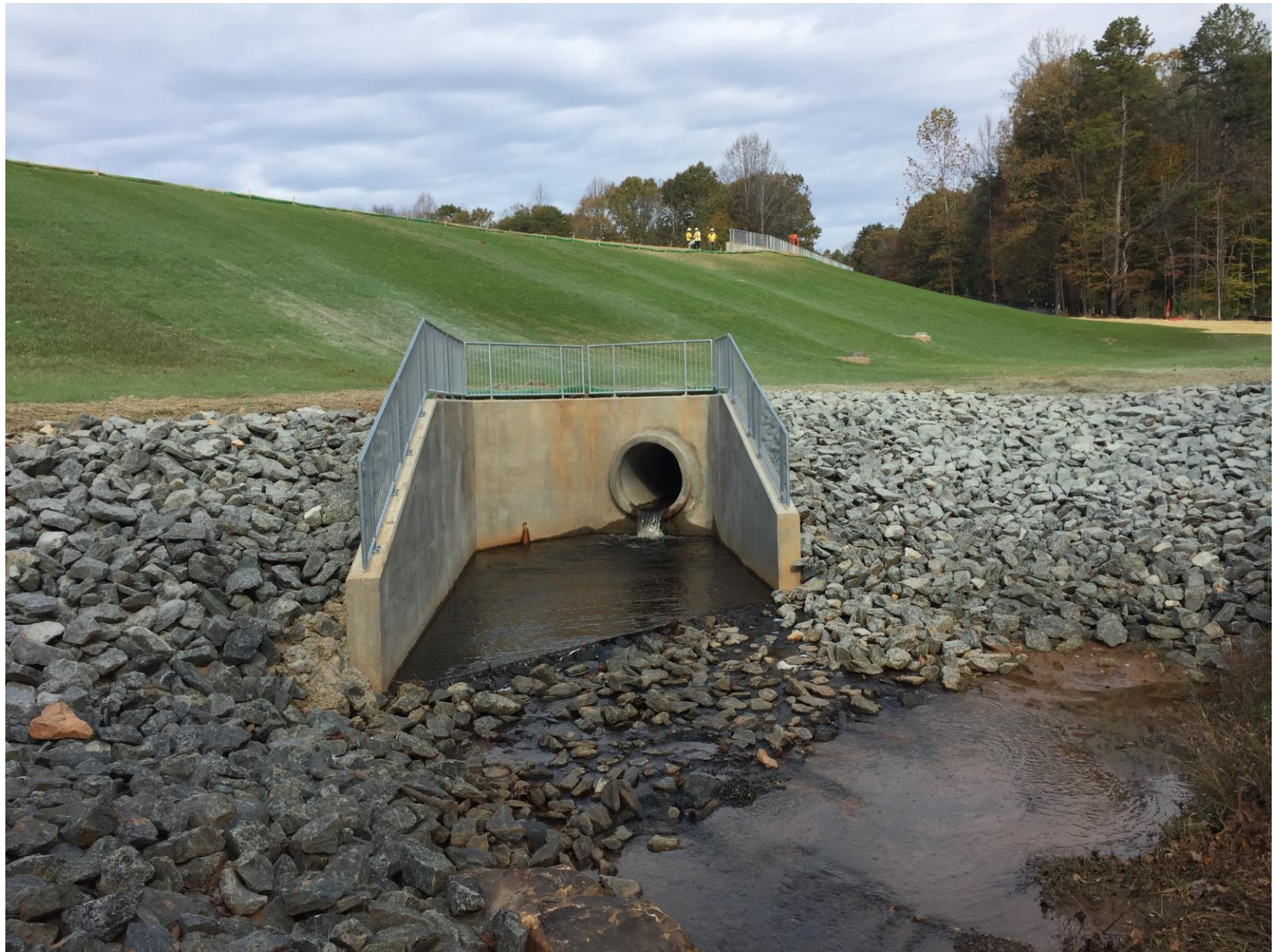
Hollymead Dam Improvements – 2018-2019
